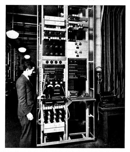
Fig. 3—Equipment for use in applying printing telegraph signals to the transatlantic radio telephone circuit at the technical operator's position.
