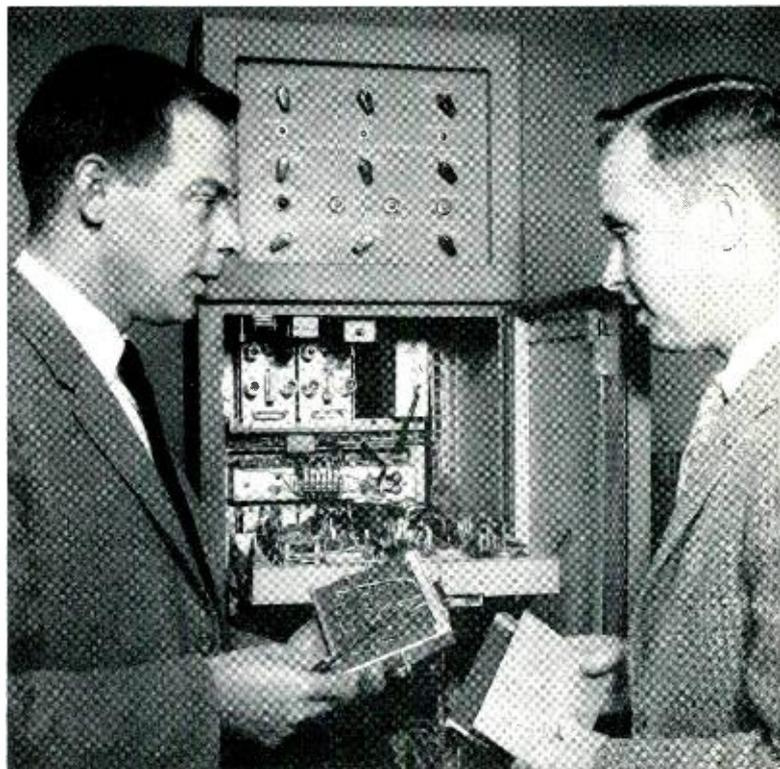
*C. C. Willhite (left) and J. W. McIntyre are examining the "square" input network of the Tracking Data Evaluator. TDE standard deviation circuits require instantaneous input voltages to be squared.*
