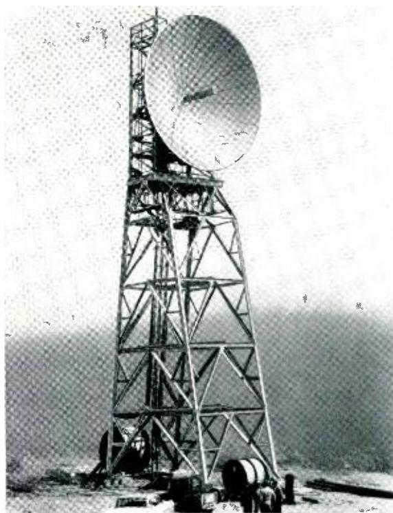
*The lateral communication system transmits one thousand watts from 30-foot parabolic antennas.*
