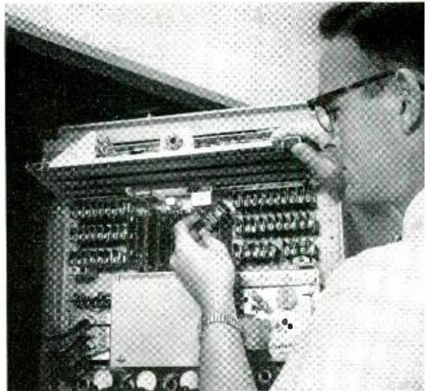
Fig. 1 — L. M. Smith examining one of many plug-in circuit units used in AN/TSQ-7 transmitter.
