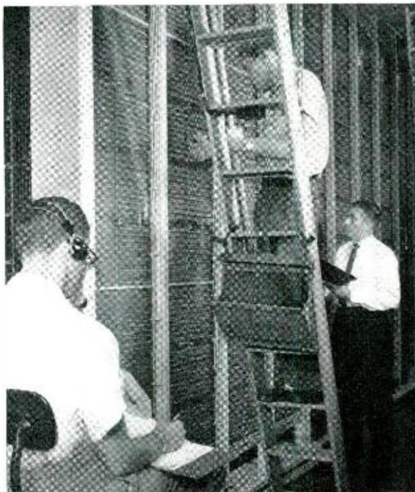
*Fig. 4—B. Pollack, left, and author check measurements on number-network frames. M. Bertelo of the New Jersey Bell Telephone Company, on ladder, makes directory number change with the new hand-squeeze grip wire-wrapping tool.*
