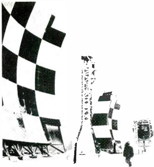
*"Beyond-the-horizon" antennas transmit and receive over distances up to 200 miles in the network.*
