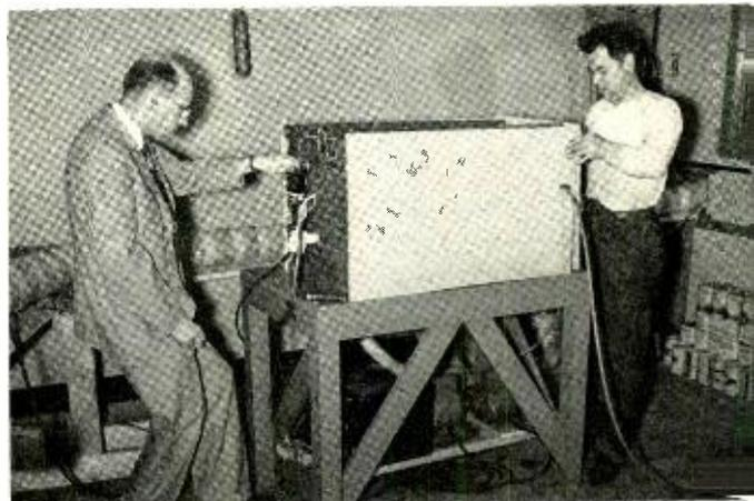
Above, R. B. Ramsey (left) adjusts the thermostatic switch in the test set-up for making measurements on a section of K cable under controlled temperature conditions. R. A. Ragan, Western Electric craftsman, is placing a cover on the refrigerant container.
