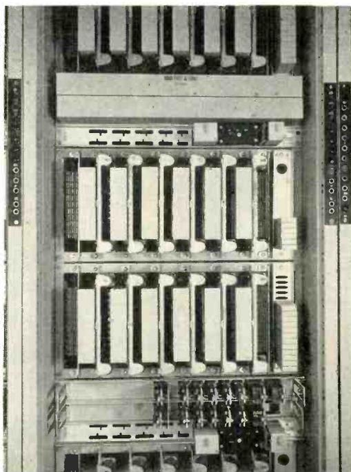
Fig. 4 (above)—On this line link connector frame, the jack strips in the face of the frame uprights are plainly evident.
