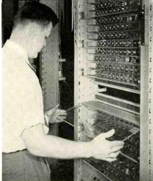
*Front view of translator and route relay frame showing method of removing front covers.*
