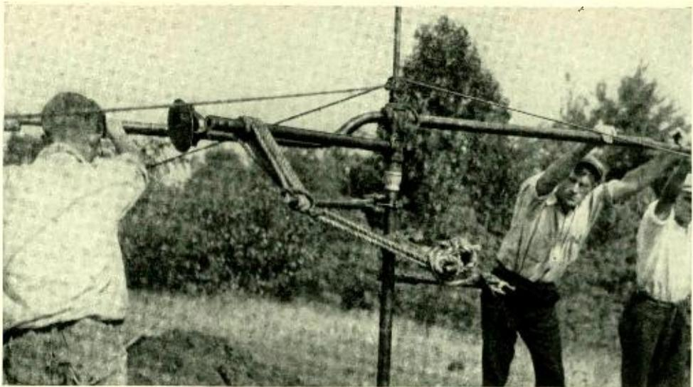
*Fig. 6—Earth anchors of the screw type used in guying poles in sand and swamp land are tested by measuring the torque required to force them into the ground*
