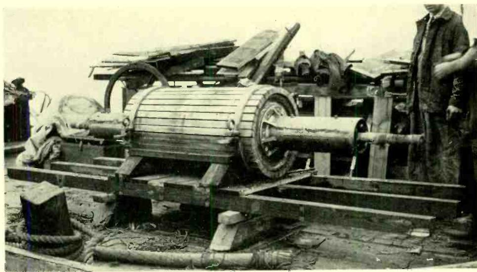
*Fig. 5—The new submarine loading coil case ready for installation*
