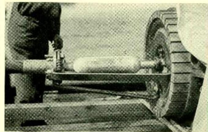
*Fig. 3—Temporary spacing bars secure the clamping rings in the proper position until after the splice has been completed*
