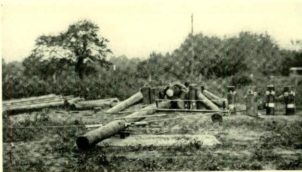
Fig. 5—Sidewalk guy fixtures, used where clearance above sidewalks is required, are tested at the Chester field laboratory by mounting them on poles supported horizontally close to the ground for convenience of measurement
