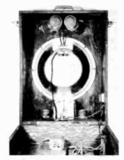
Fig. 4. Experimental assembly of 12" cone and University Model 4402, with dividing network and impedancematching input transformer.
