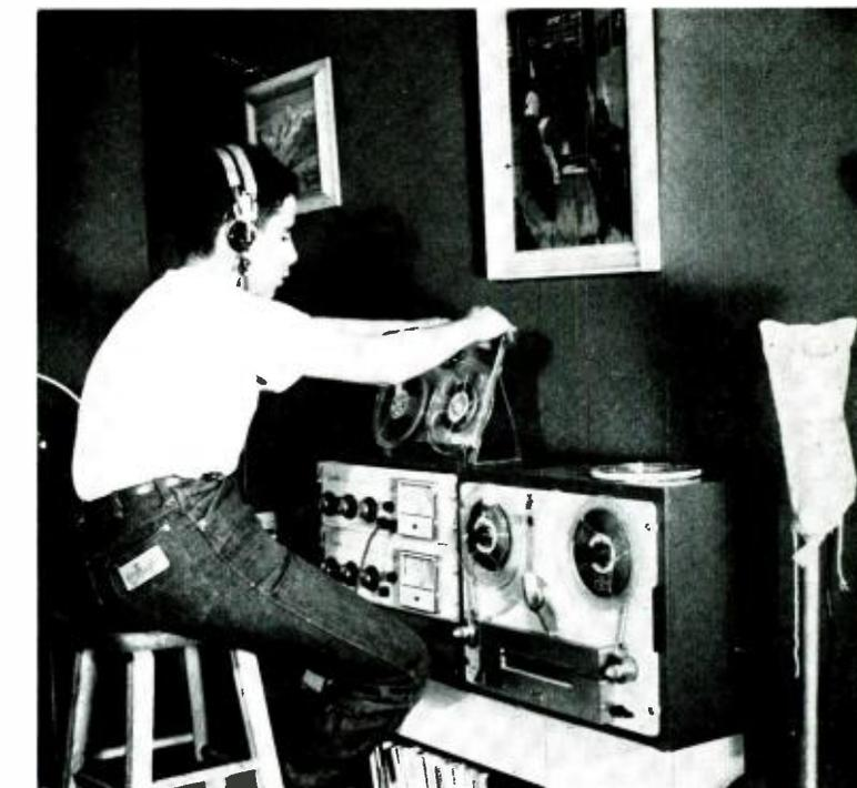
Inserting Pauses in Continuous Speech Records. Output of Viking goes to Channel 1 input of Concertone; latter runs continuously, while Viking is stopped at the end of each sentence or phrase for the desired pause.
