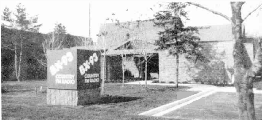
Rick Richardson, President of Middlesex Broadcasters, can be proud of his new facility considered one of the most modern and up-to-date listening posts in North America.
