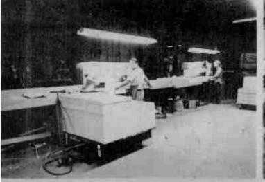
Automatic paper cutters for trimming of printed jacket flaps.
