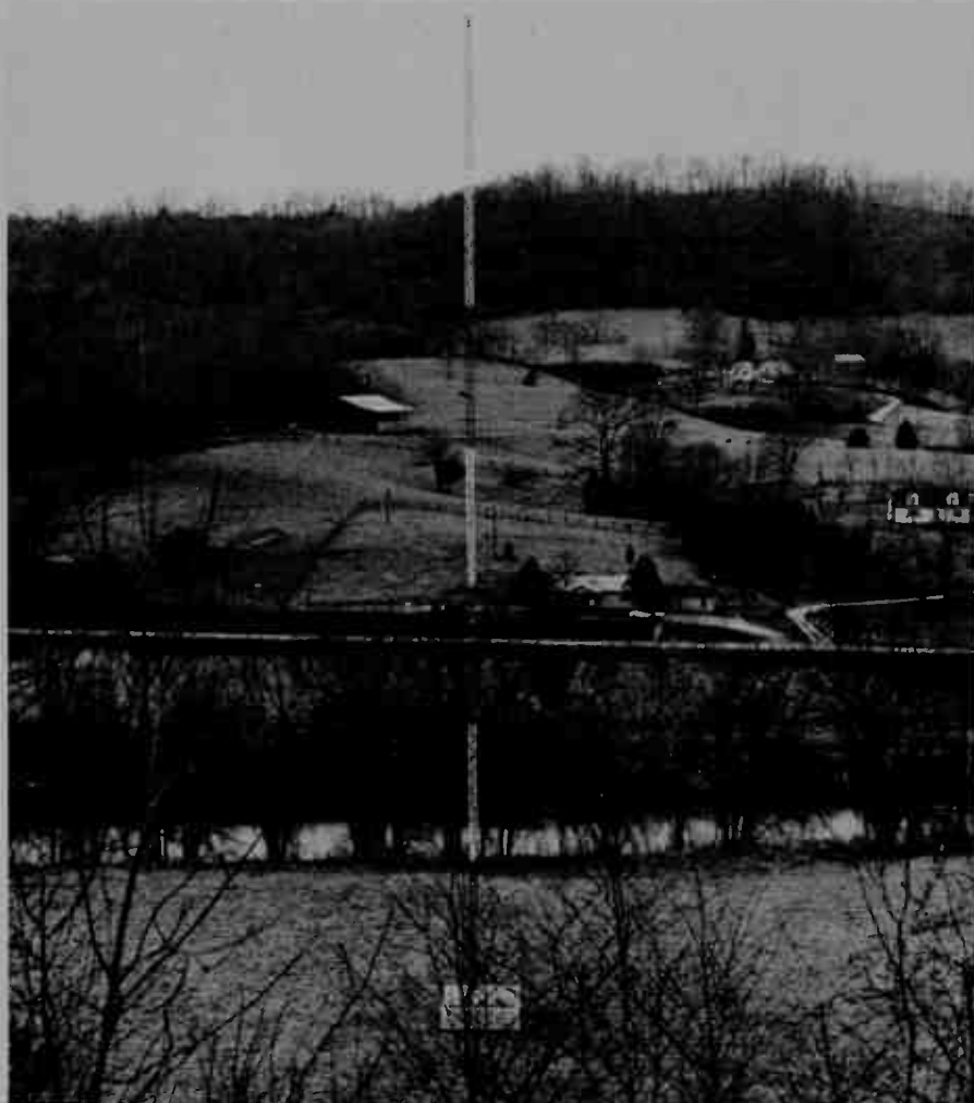
WEKG's 215-foot tower; 1,000 watts power.
