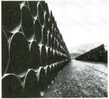
It took over one-half million tons of steel to make the 798 miles of pipe for the project. The sections are 40' and 60' long, 48" in diameter.
