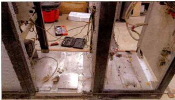
Heavy Transformers Removed
