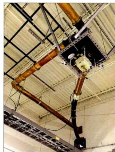
Figure 8. The repaired RF switch with plexiglass guard. Also shown are the connections to the main and spare transmission line.
