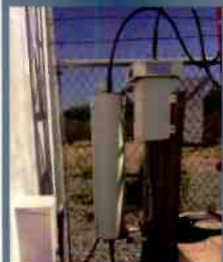
Full line of Isocoils for co-locating 1 or more FM Translators on AM tower
