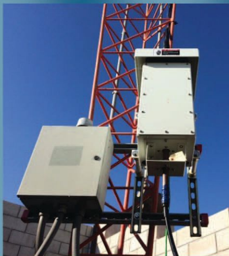
Model FMC-1.5 Isocoupler for low-loss isolation solution
