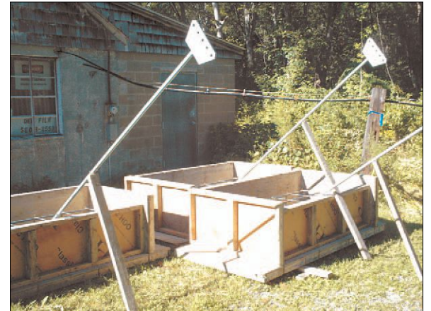
Guy wire anchors ready for concrete.
