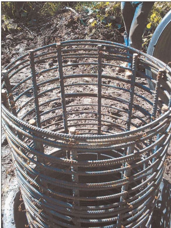
Tower Base Rebar
