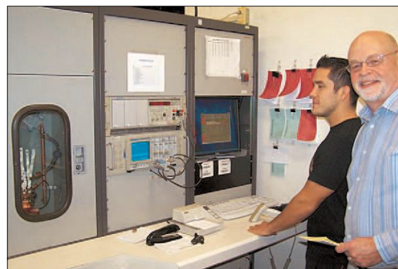
John Canevari and Rafael Alcalá, test console operator, check test results on tube.
