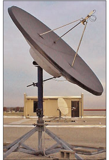
Photo-1: A 3.8m Comtech Dish with a DAWNco cover.
