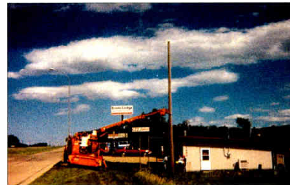
An emergency antenna right on site.
