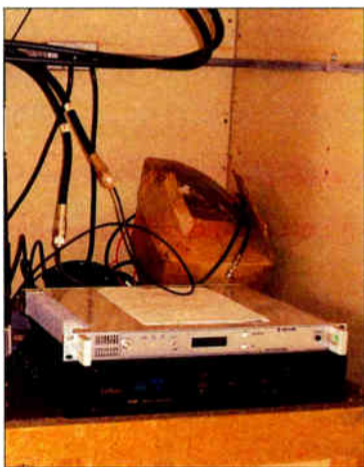
Ungrounded, the transmitter and receiver were stacked on the counter – rubber feet and all.
