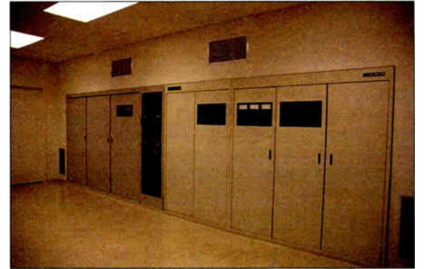
The 3DX50 Main and DX50 Aux transmitters fit in the place where the 50HG used to sit.
