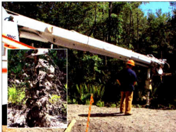
Setting the counterpoise poles was handled by one man, but was a messy job.
