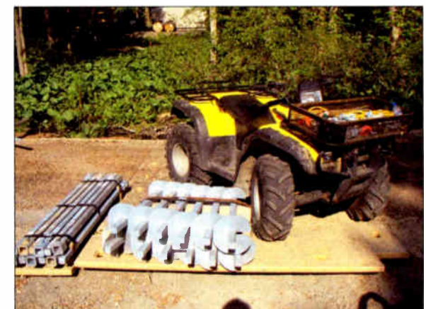
Helical anchors were used to overcome the difficult soil conditions
