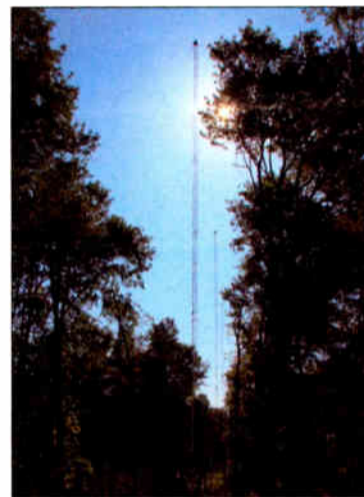
The completed array, neatly slipped into the swamp with as much clearing as was allowed.
