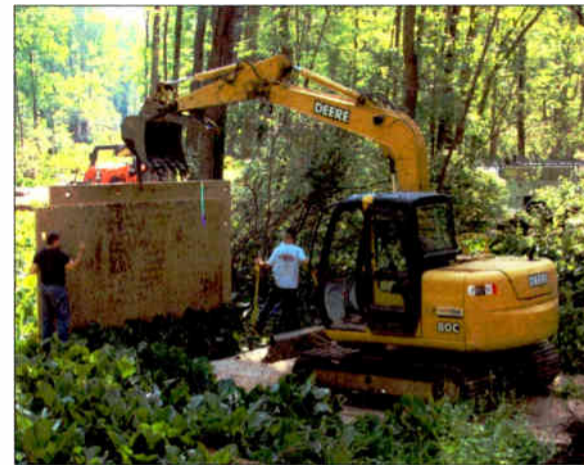
To protect the swamp, some 100 large mats were installed temporarily.
