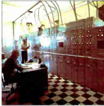
A 3 kW Westinghouse transmitter in Canada.
