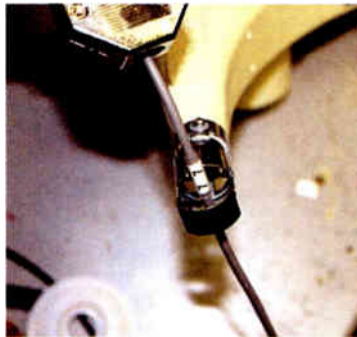
Using clear heat shrink makes identification of the wiring much easier.
