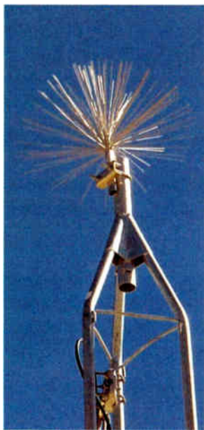
Multiple points can dissipate larger charges.
