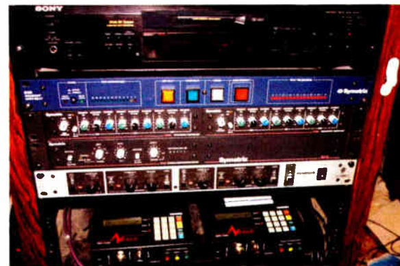
Telephone and audio control units.
