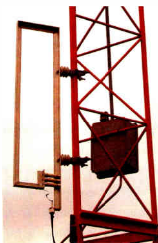
Typical single turn unshielded sample loop.
