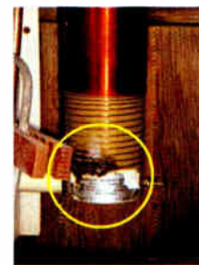
An Ex-Static Drain Choke
