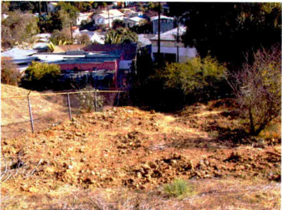
Some of the dirt left by a less than neighborly neighbor. The Building and Safety inspector's visit finally put a stop to it.
