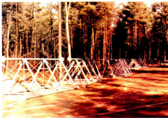
A closer look at a “mass of triangles.” Recently assembled seven foot face, by twenty foot high, triangular sections await stacking.”
