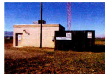
A nice and properly fenced site.
