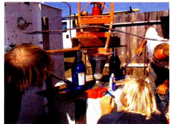
Slowly jacking the tower off its insulator.
