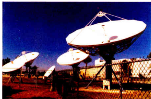
Lightning Protection on Dishes
