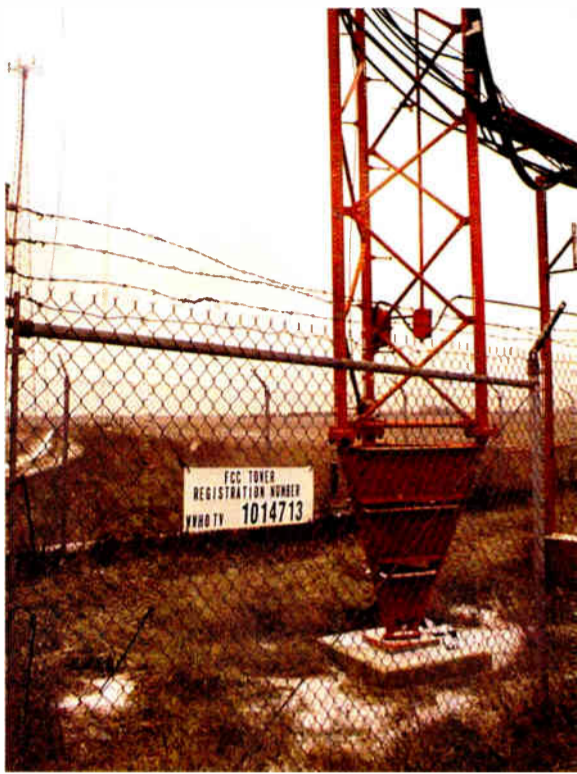
ASR signs mounted on chain link fences can be easily vandalized.
