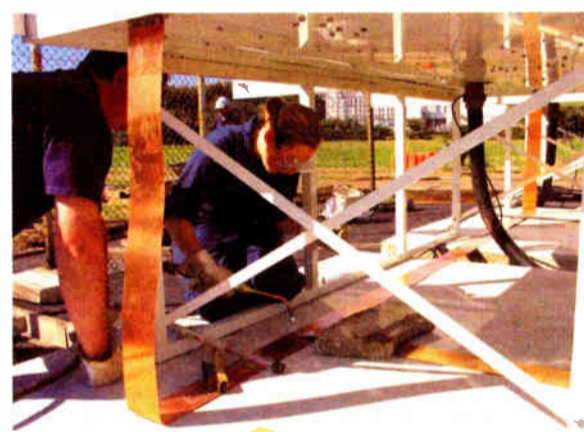
Ed Trombley working on a Directional Installation in Japan.
