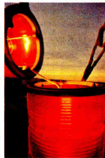
An open beacon fixture. Note the bulbs are lit.
