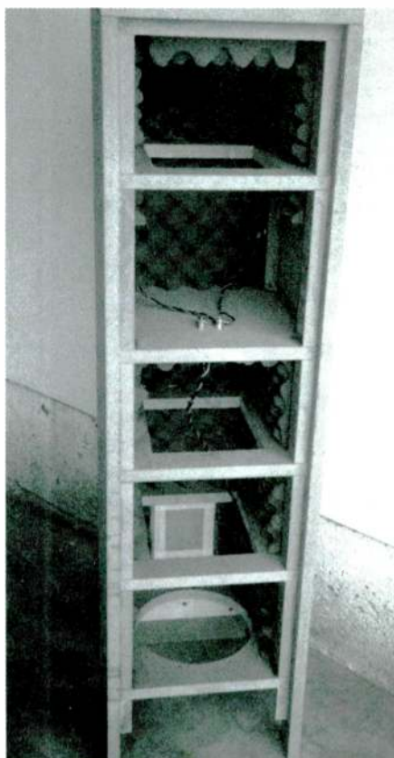
PHOTO 11: Foam and wiring installed in cabinet.
