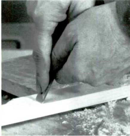
PHOTO 16: Using a chisel as a scraper.
