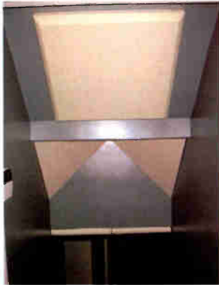
A two-inch thick, 24 X 24-inch beveled-edged panel and two Cumulus mid-bass traps perform quite well in the stairwell to the room from the house's main level.
