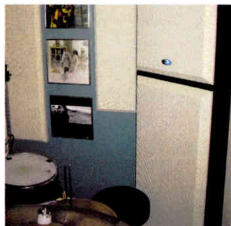
L to R: Two two-inch thick, 12 X 48-inch beveled-edged panels and two MaxTraps, stacked, create the front left corner of the room, which is currently set up for live drum tracking.
