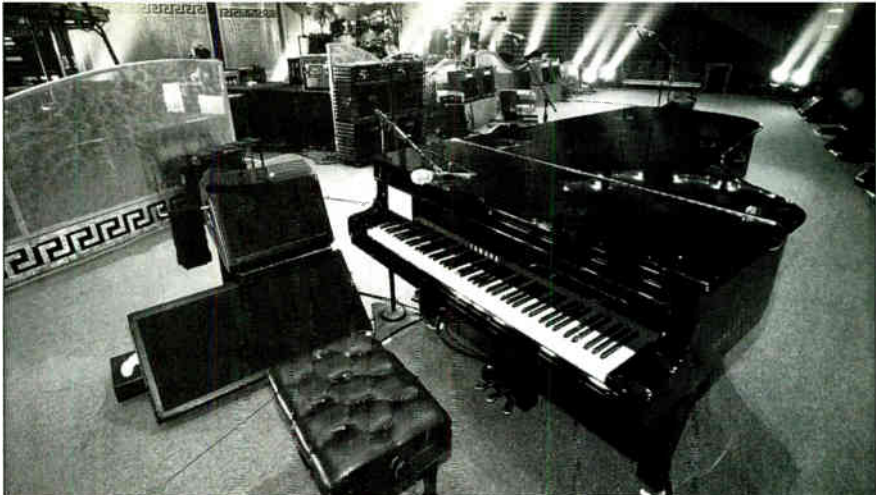
Elton John's stage monitor setup includes stereo pairs of Clair 12AMs and 2x15 wedges (the downstage units, not shown, sit side by side to preserve sight lines). Screen at upstage edge of piano is for a TelePrompTer.
