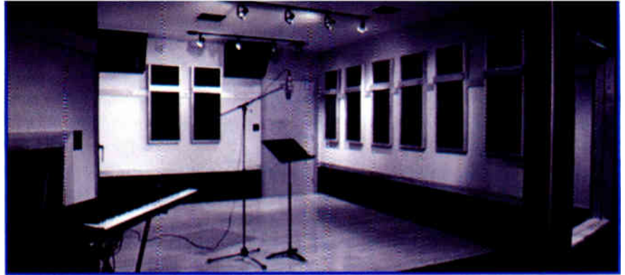
Pilchner Schoustal Architectural Acoustics designed this new facility for Angel Mountain Productions (formerly known as Sloyer Sound) in Bethlehem, Penn. The floating live room was built with moveable panels that allow the recording space to be adjusted for a sound from dead to extremely bright. The control room is equipped with a 40-channel Soundcraft DC2020 console, 24-tracks of Sony PCM-800, and monitors by Quedest, Genelec and Tannoy.
