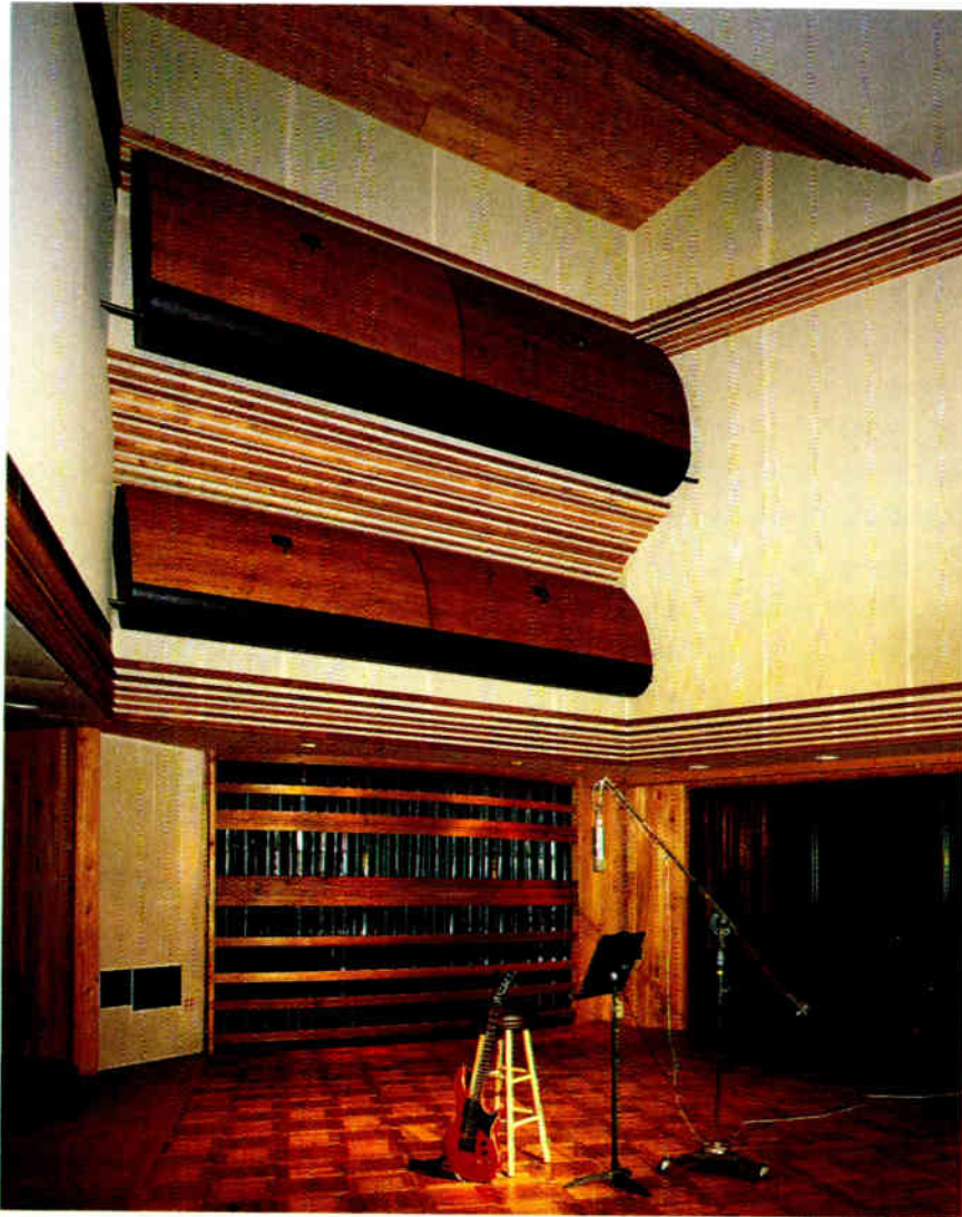
The John Storyk-designed downstairs East Wing studio at Criteria boasts a 40,000 cubic foot recording room with 27-foot ceilings. Motorized wall panels can be remotely adjusted to vary acoustics.
