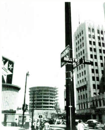
The Capitol tower under construction in 1955.
