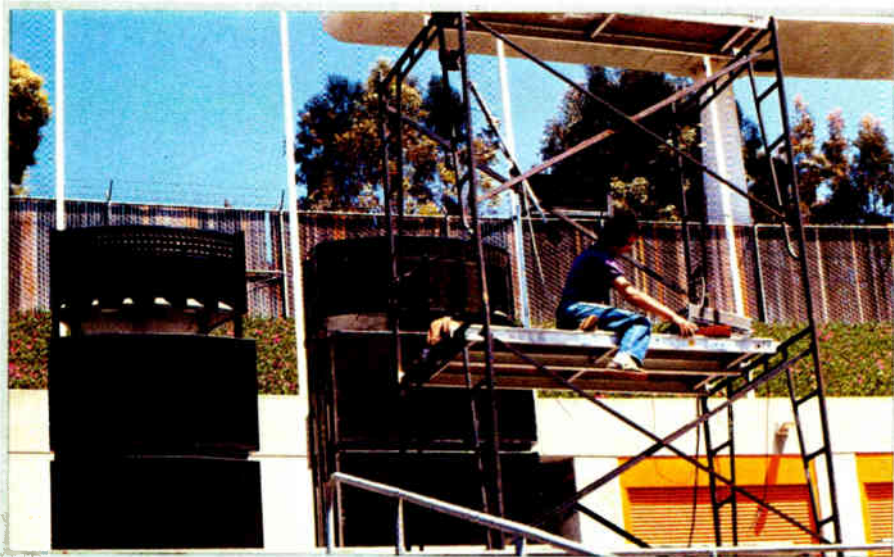
Technician runs A/B tests of HMS-12 and JM-10 systems.
