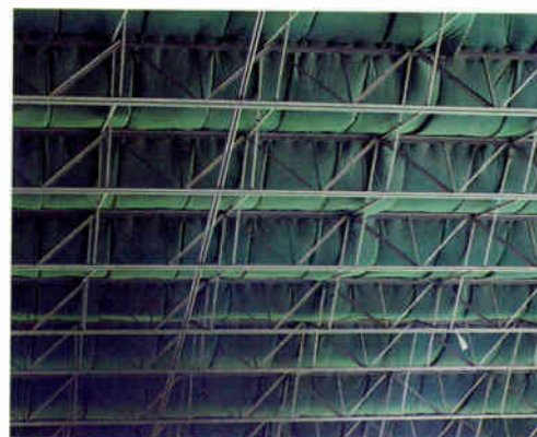
Acoustical Solutions' Sonex (covered with material so that it is unseen) was used to soften up the shell.
