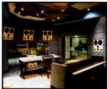
Control room B, with Control 24 worksurface
