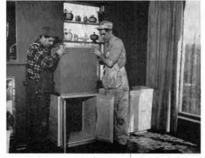
Fig. 9. Final construction of the cabinets was completed on the job. Here one of the enclosures is being lowered into the speaker section of the right-hand cabinet
