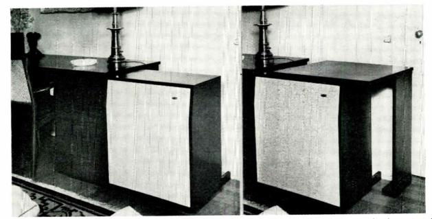
Figs. 4 and 5. The legs were removed from each speaker, a base substituted to match the 30-in. height of the desk, and this closure piece added
