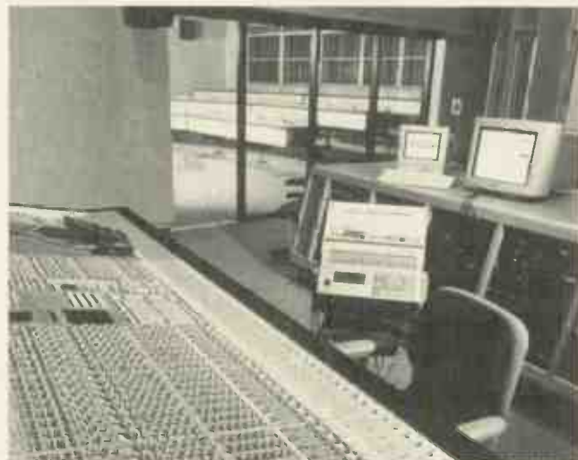
SSL console located in MTSU's $15 million Mass Communication building
