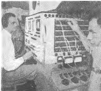
This view shows the video monitors (left) and the audio monitors with plane-ground "cue" circuits on the right.
