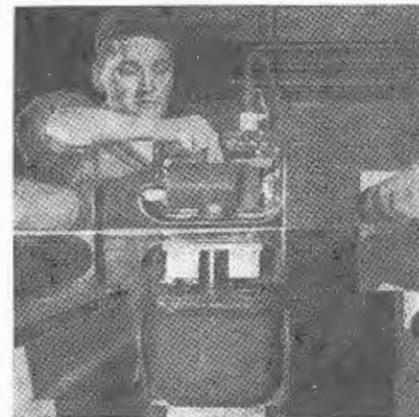
Both x-ray tubes and their transformers are mounted in a single, oil-filled cast head. In this installation, the steel strip is shown passing between the lower x-ray generator and the pickup photomultiplier above it.
