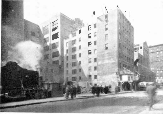
WORK IS WELL UNDER WAY
