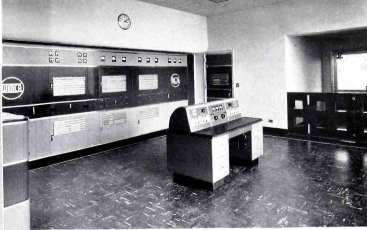
▲ The streamlined RCA 5-DX, 5 KW Transmitter, installed at WMCA with its associated control desk.
