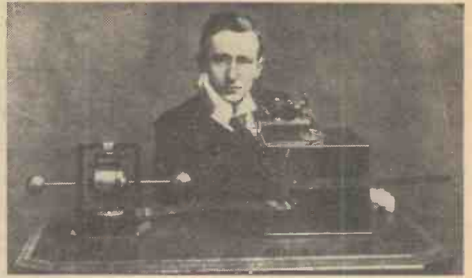
Marconi, with original apparatus—Hertz oscillator and coherer receiver—which he brought from Italy. (Photograph taken in 1896.)
