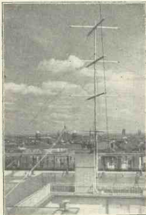
An experimental ultra-short-wave aerial erected upon the Europahaus, Berlin
