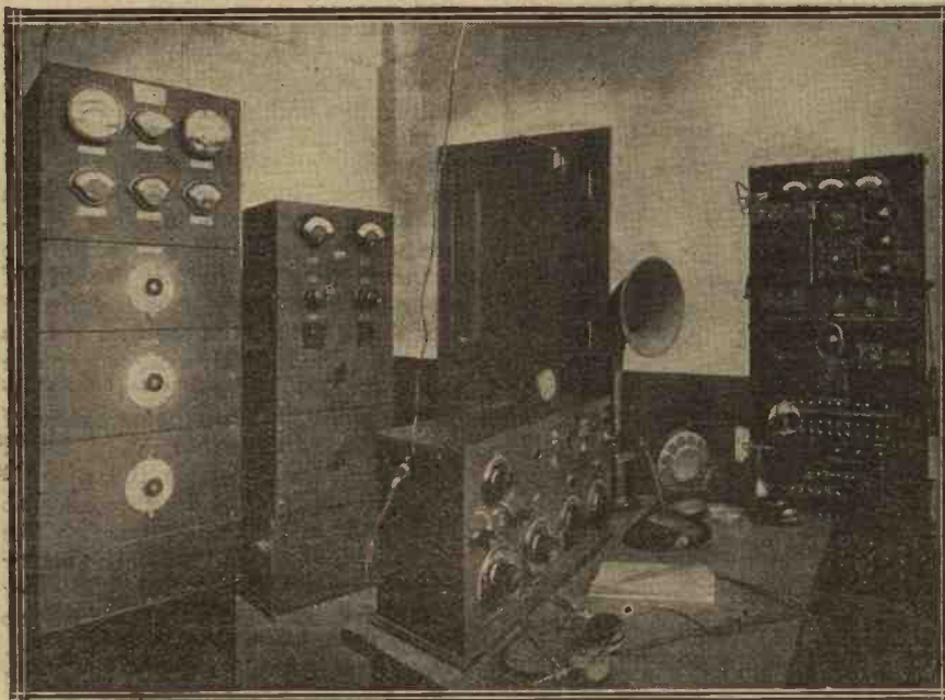
The control room at station WAHG, Richmond Hill, New York.
