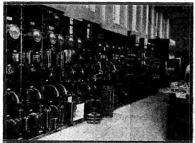
The low-tension switchboard in the valve room at the Rugby wireless station.
