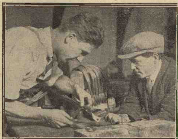
Taping the ends of the inductance windings at the Post Office Wireless Station at Hillmorton.
