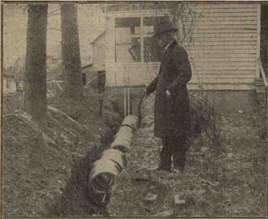
A buried aerial has been found fairly effective in reducing the amount of atmospheric interference in the receiver.
