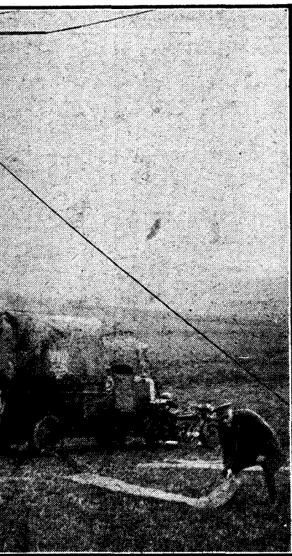
Earth mats for a mobile wireless station.
